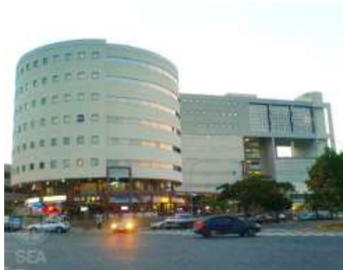
Figura 25: Imagen del C.C Reda Building.
