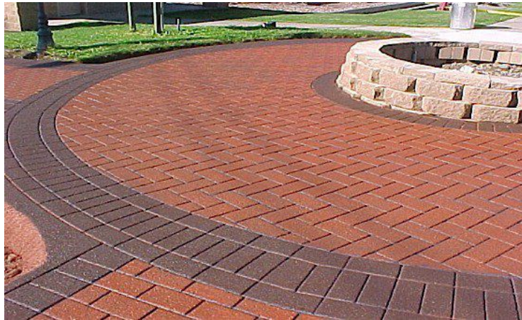
Figura 24 Asfalto Estampado https://www.google.co.ve/search?client=firefox-b&biw=1366&bih=635&tbm=isch&sa=1&q=asfalto+estampado&oq=asfalto+estampado&gs_l=img.3...228212.231122.0.231381.0.0.0.0.0.0.0.0...0...1.1.64.img..0.0.0.GMIBny4Cu1M#imgsrc=L5igfJesK10yFM:
