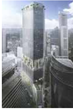
Figura 6. Fachada 88 Market Street.
