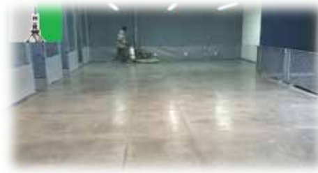
Figura 26: Piso de concreto pulido fuente: https://mx.depositphotos.com/128126330/stock-photo-concrete-floor-white-dirty-old.html (2018)
