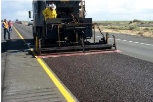
Figura 78: Slurry seal
