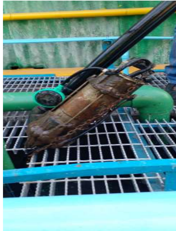
Bomba sumergible
