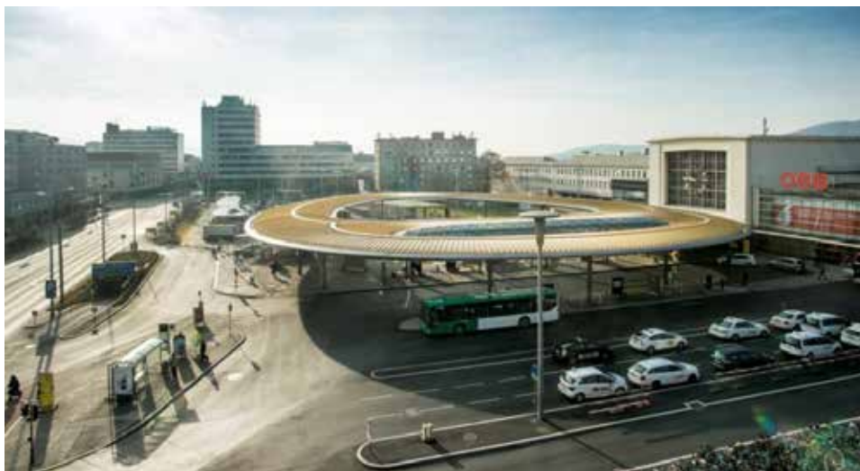
Figura 3: Graz Main Station Local Transport Hub.
