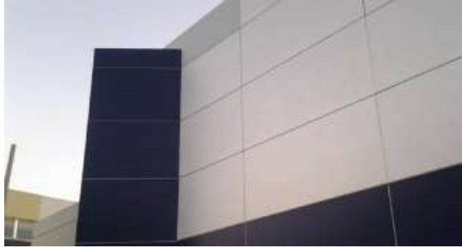
Figura 8: Paneles de Alucobond
