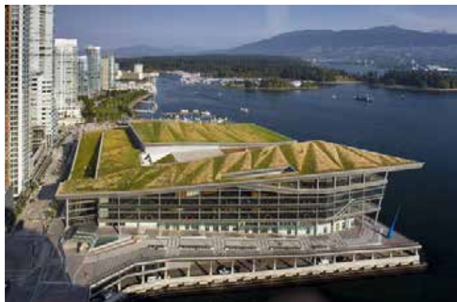
Figura N°40 Techo verde Vancouver Convention Center
