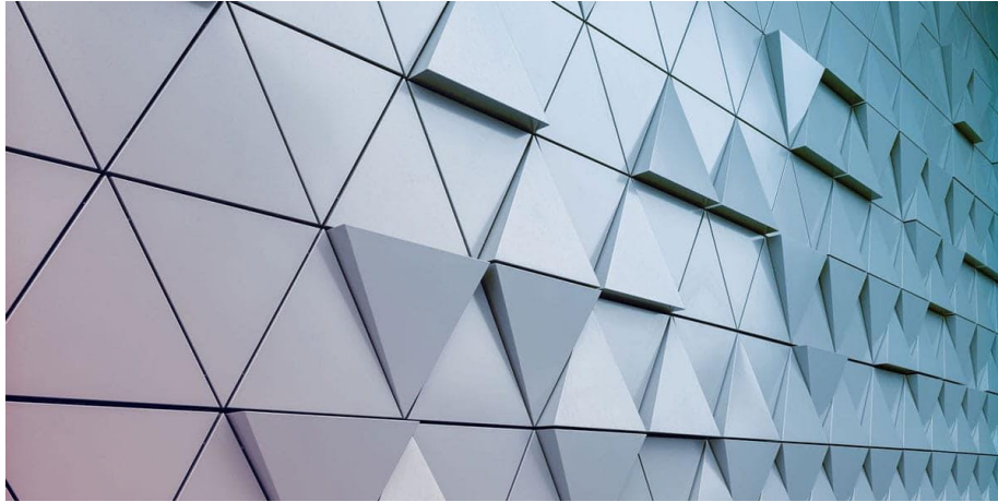
Figura 25, Paneles de alucobond.
