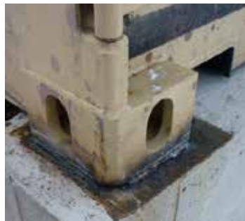
Figura 39. Cantonera soldada al contenedor. http://www.tincancabin.com/wp-content/uploads/2011/01/Welding1.jpg (2017).
