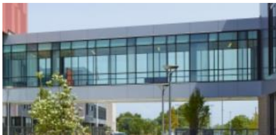
Figura 24. Materiales para Puente. Fuente: https://cornergreer.com/projects/joplin-high-school-franklin-technology-center (2015).
