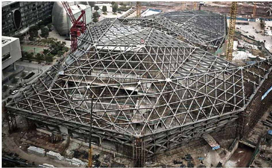
Figura 120. Zaha Hadid, malla estructural(2015) fuente: https://oscartenreiro.files.wordpress.com/2015/02/19-guangzhou-opera-house-en-construccion-de-zaha-hadid.jpg
