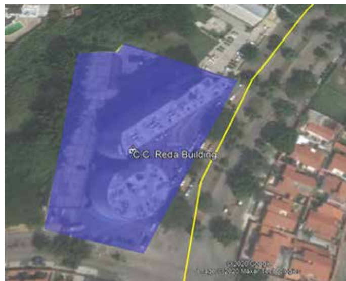
Figura 73. C.C. Reda Building.
