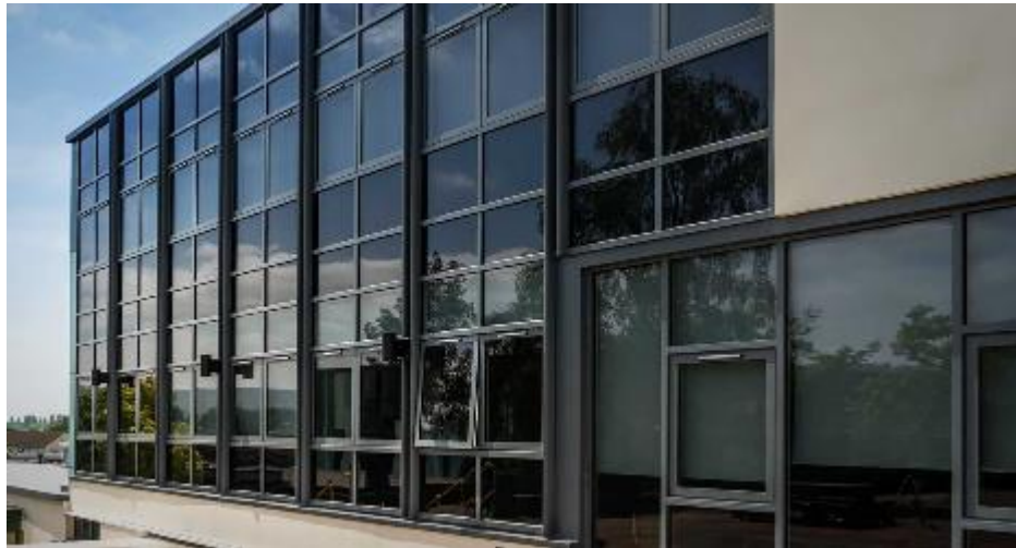
Figura 35. Modelo de Muro Cortina. Fuente: http://www.avdon.co.uk/wp-content/uploads/2017/07/grey-aluminium-curtain-wall.jpg (2018)
