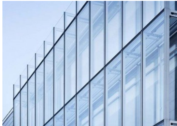
Figura 50 Curtain wall. Fuente: https://www.designingbuildings.co.uk/wiki/Curtain_wall_systems .(2017).
