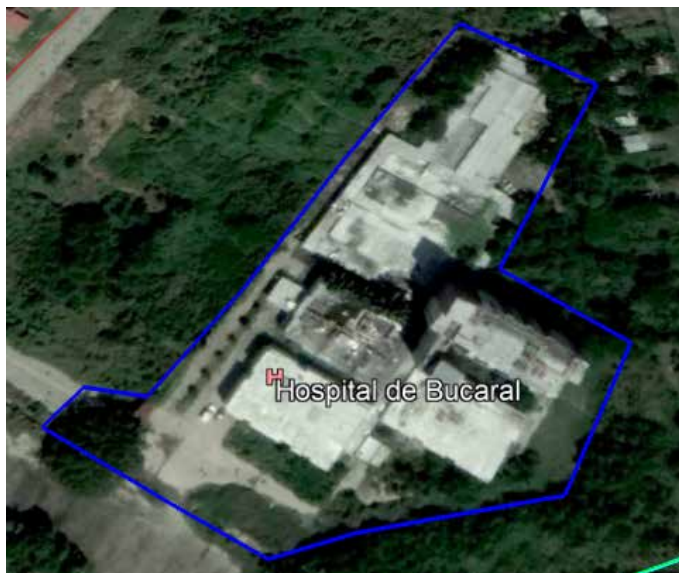
Figura 10: Vista satelital Hospital de Bucaral
