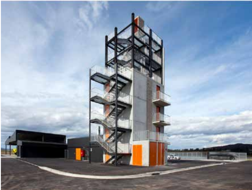
Figura 4: ACT Emergency Services Agency OTC, Hume, Australia, 2011 Fuente: https://www.plataformaarquitectura.cl/cl
