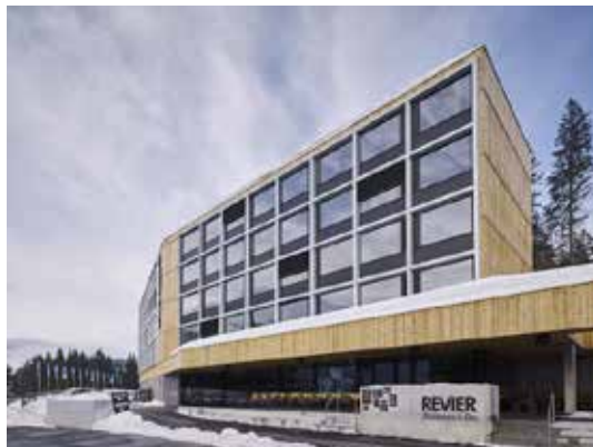
Figura 1. Fachada principal del Hotel Revier.
