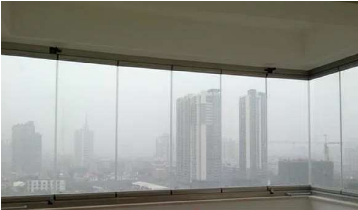
Figura 60. Ventanas desplegadas deslizantes sin marco. Fuente: http://www.terraceglazing.com/balcony-glazing/famous-balcony-aluminum-and-glass-frameless.html (2022)
