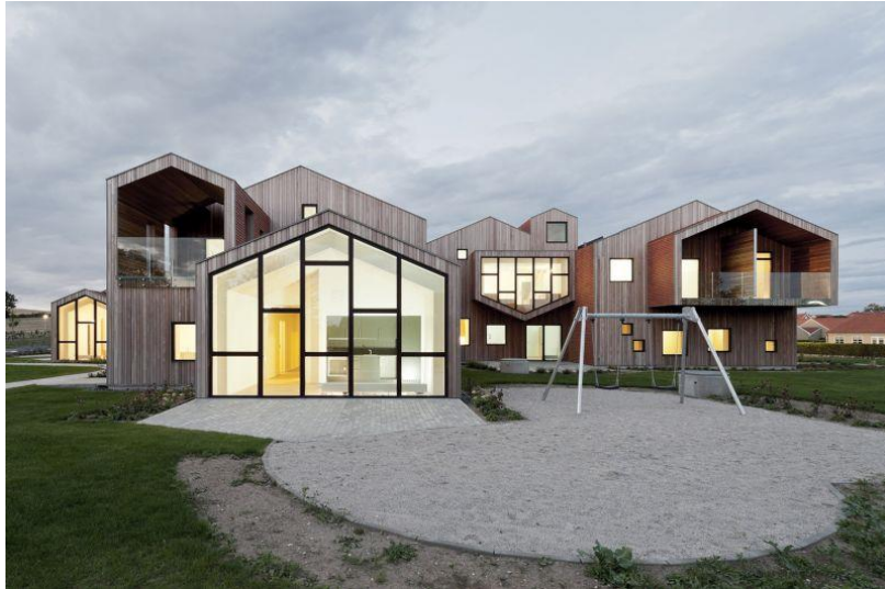
Figura 8, Fachada Posterior, https://arquitecturayempresa.es (2019).
