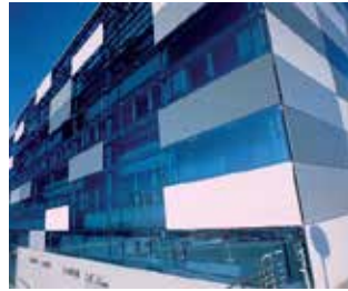
Quadroclad – Hunter Douglas. Fuente: http://www.archdaily.com/69559/quadroclad%25e2%2584%25a2-glass-facade-panels-hunter-douglas-contract/orchard02(2017)
