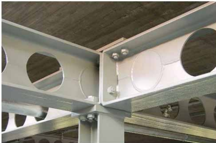
Figura 50: Vigas Alveolares. Fuente: http://sections.arcelormittal.com/fileadmin/redaction/4-Library/1-Sales_programme_Brochures/ACB/ACB_ES.pdf
