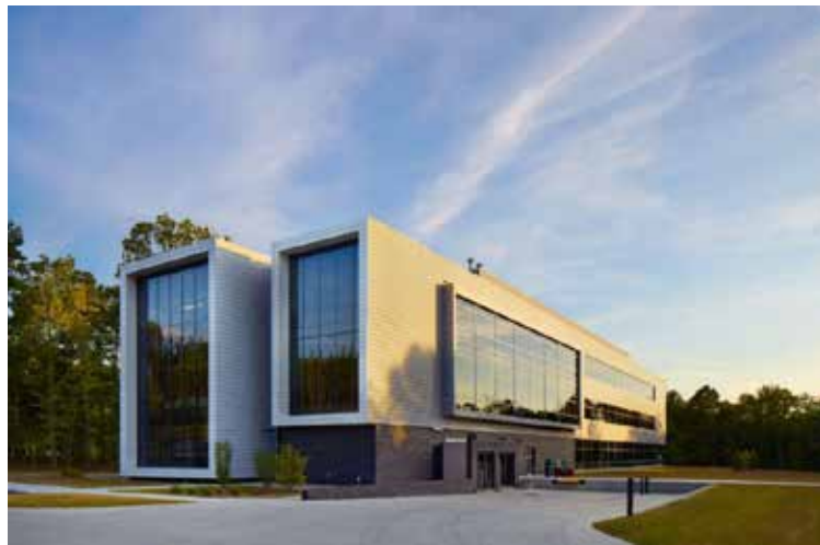
Figura 2. Bioprocess Innovation Center / Clark Nexsen Fuente, https://www.archdaily.com/879329/bioprocess-innovation-center-clark-nexsen?ad_source=search&ad_medium=search_result_projects (2017)
